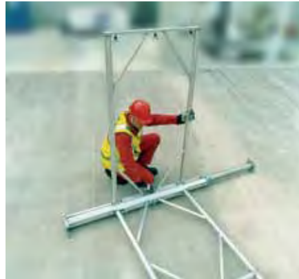
2. Connect ledger frame vertically to leg.
