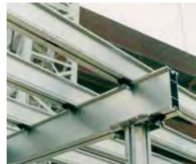
Headplate to beam fixing
