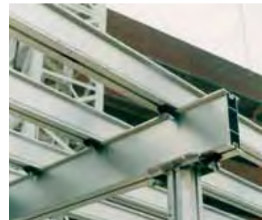
Headplate to beam fixing
