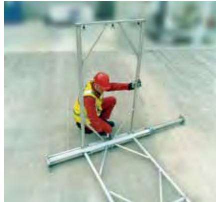
2. Connect ledger frame vertically to leg.
