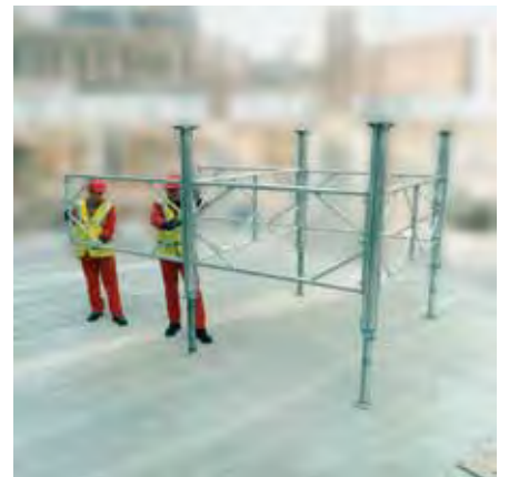
6. Now add additional frames and legs to form Megashore support structure.
