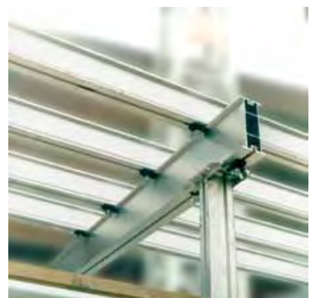
9. Position secondary beams and fix with a Megashore clamp at each intersection with a primary beam. Structure is now ready for fixing of plywood.
