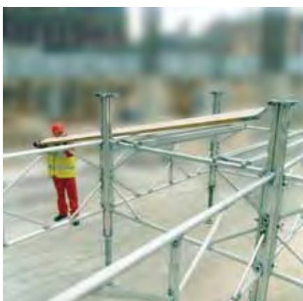
7. Place intermediate transoms and scaffold boards in position for fixing of aluminium beams.
